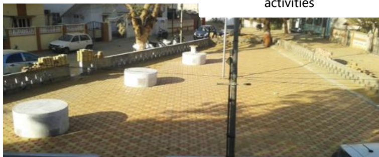
Flood control through GW recharge for a housing colony
